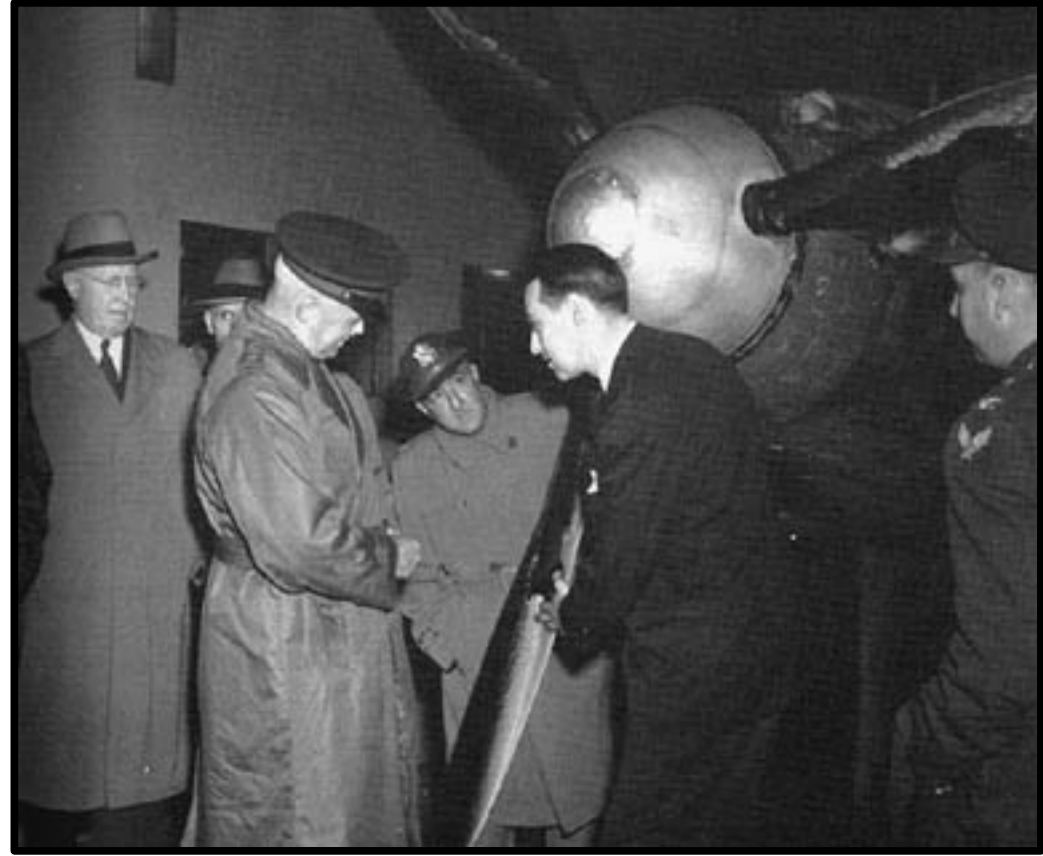
Wilson Hunter, the Head of the Icing Research Section is shown demonstrating the dangerous icing of the propellers of a P-39 after a wind tunnel test. General Arnold (left) and George Lewis (far left).
